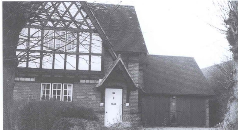
A recessed garage with harmonious roof pitch and separate doors breaking up the side wall.
